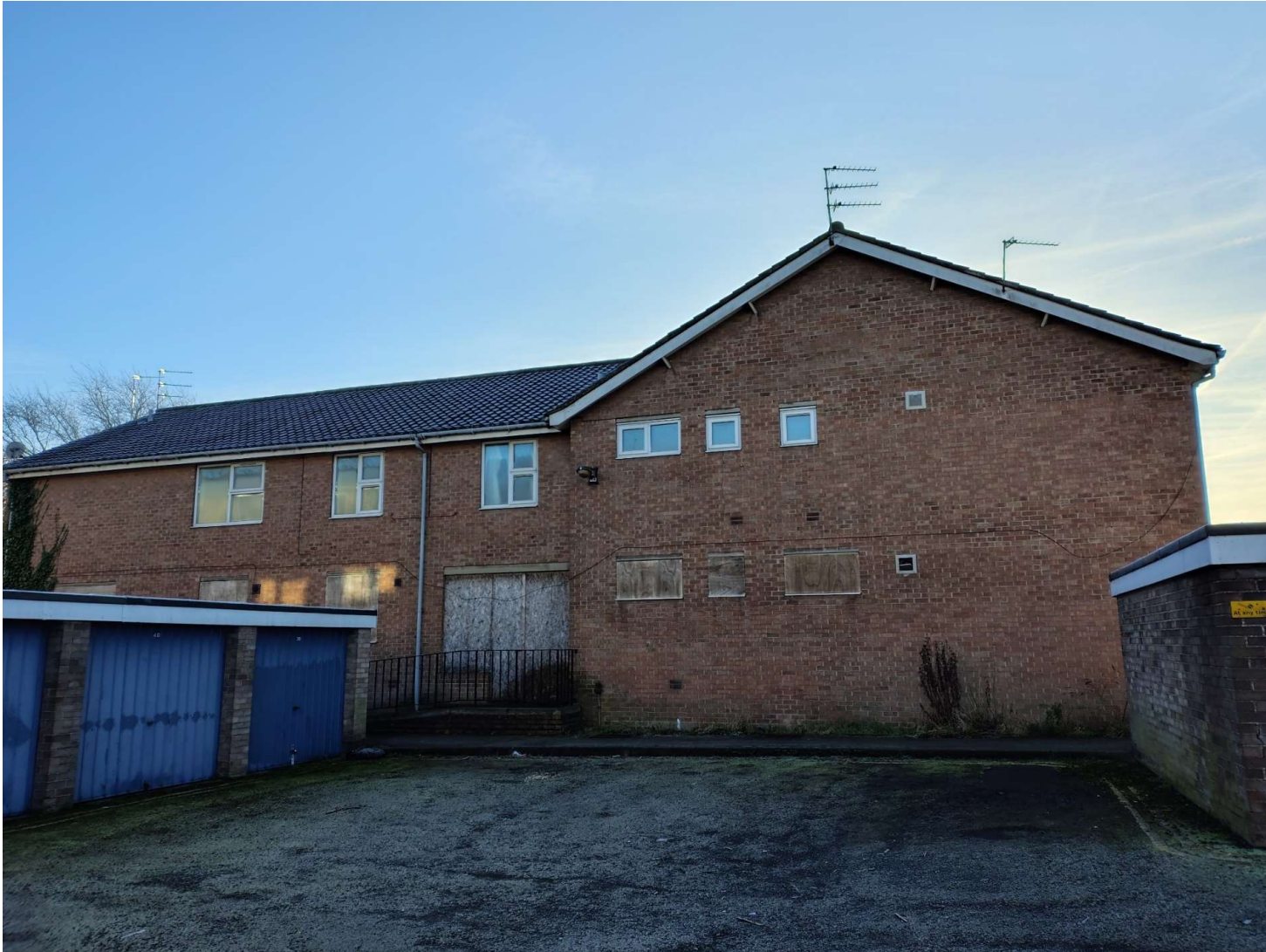
Site Photograph Willow House as viewed from North
